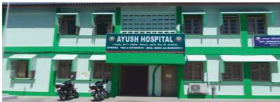
Construction of Integrated Ayush Hospital at Port Blair, Andaman & Nicobar Islands
