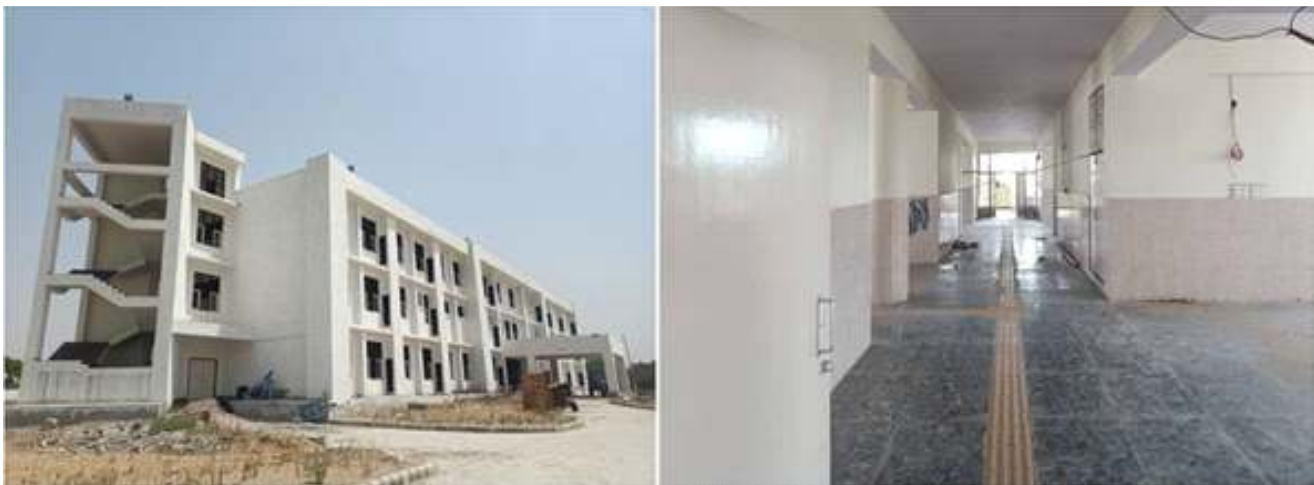
Construction of Integrated Ayush Hospital, Mayyer, Hisar, Haryana
