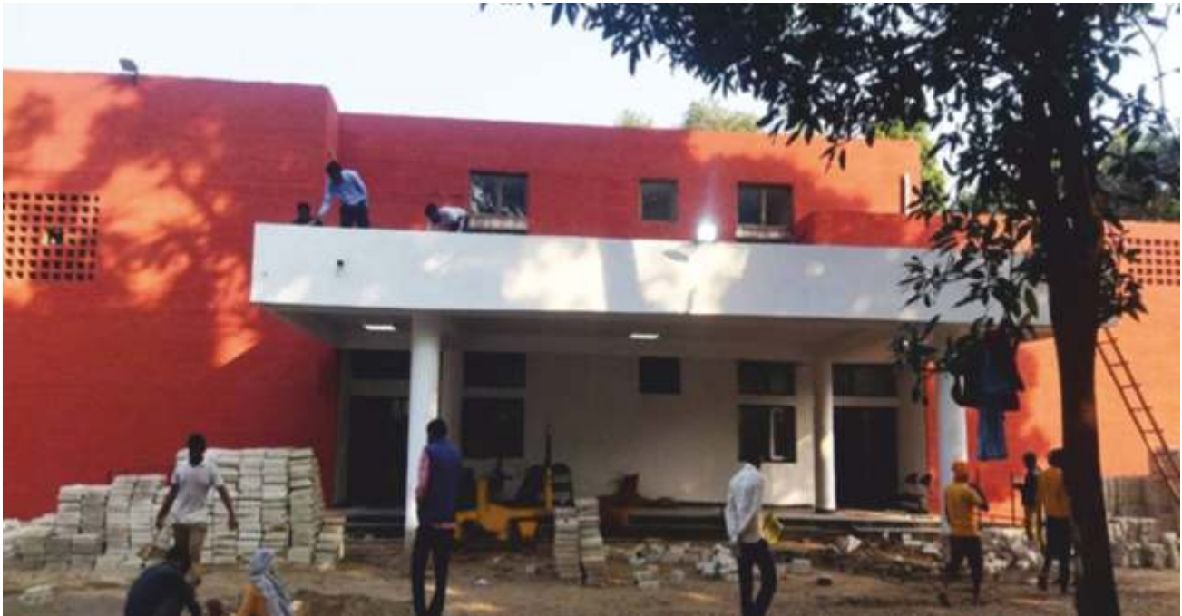
Construction of Integrated Ayush Hospital at Chandigarh
