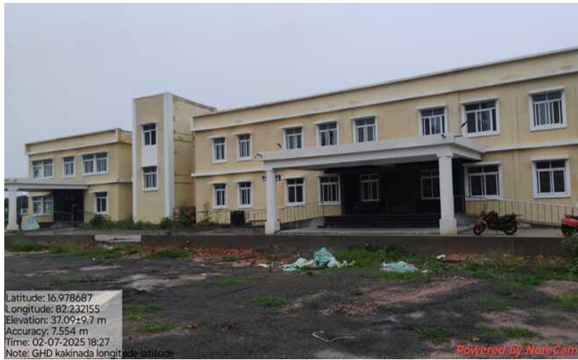
50 bedded Integrated Ayush Hospital, Kakinada, Andhra Pradesh
