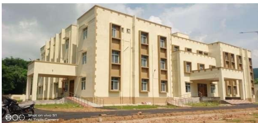
50 bedded Integrated Ayush Hospital, Visakhapatnam, Andhra Pradesh
