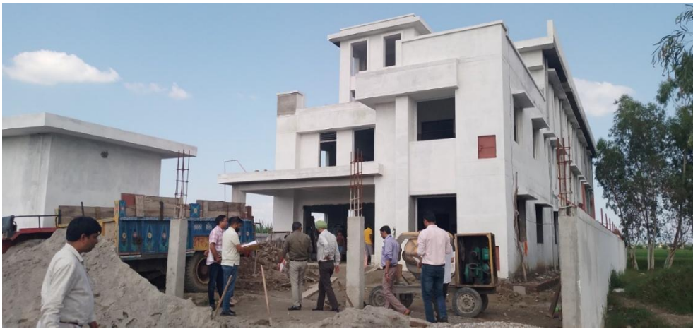
Construction of Integrated Ayush Hospital at Pathri, Haridwar, Uttarakhand
