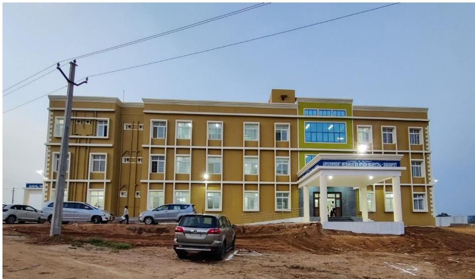
Construction of 50 bedded Integrated Ayush Hospital, Siddhipet, Telangana
