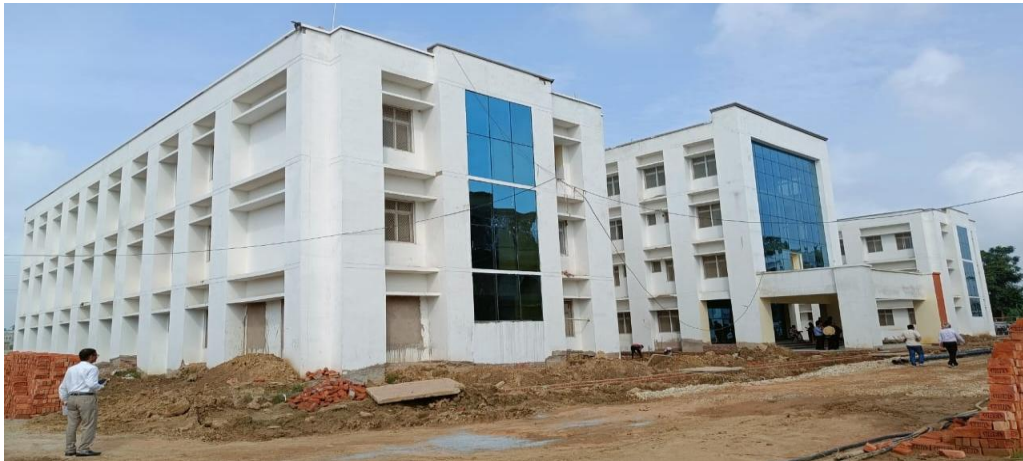
Construction of new Government Ayurveda College, Ayudhya, Uttar Pradesh
